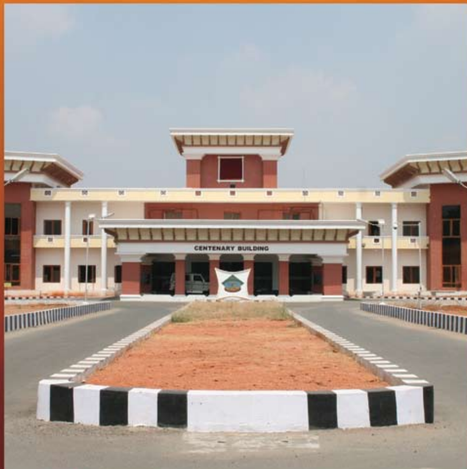
TNAU Centenary building - Inaugurated on October 27, 2009
